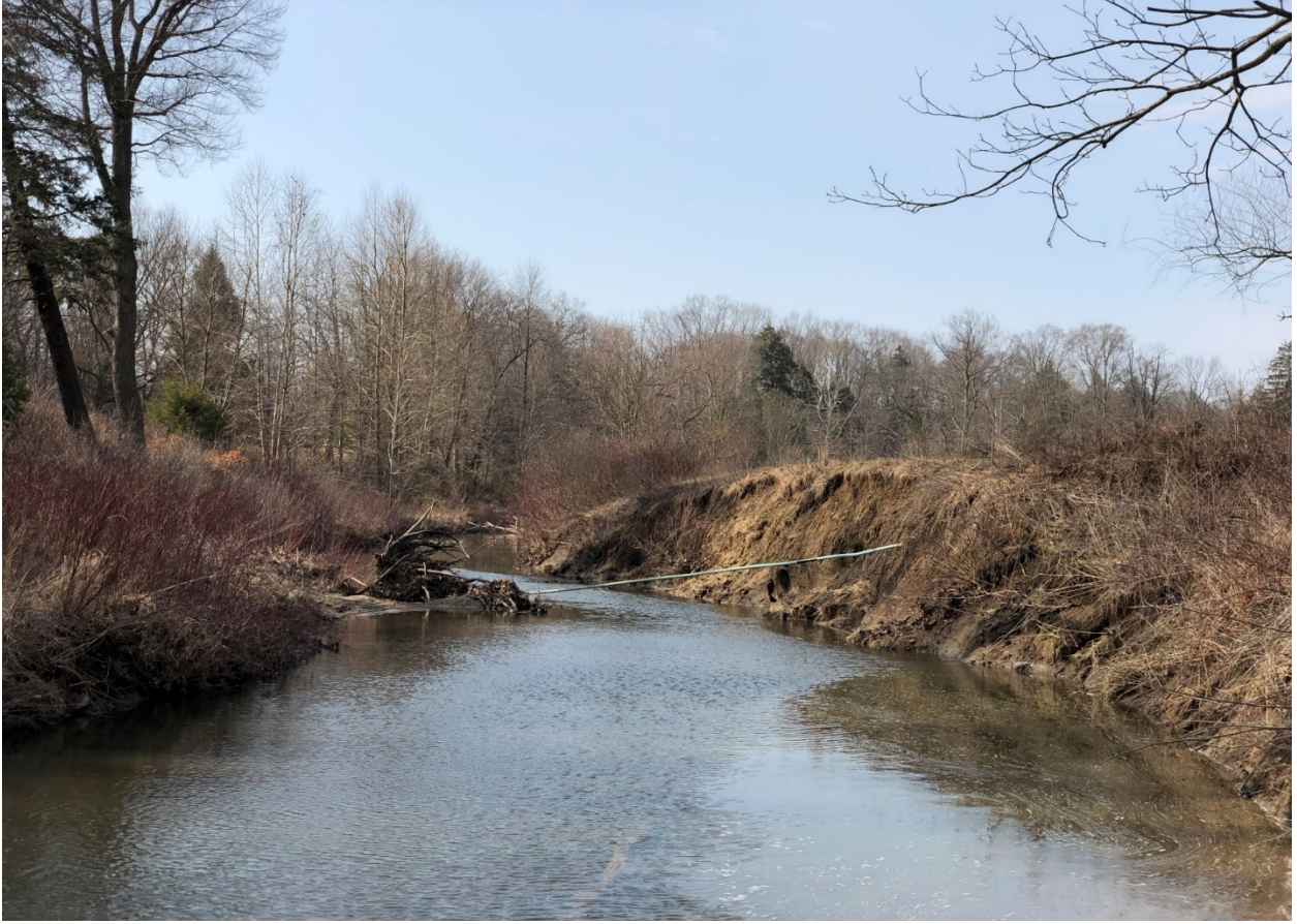
Figure 2 Smith Creek experiencing significant erosion throughout Centerville Mills (2018)
