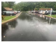
Rain travels between the joints of permeable pavers into layers of underlying stone. Some of this water soaks into the ground beneath the stone, and some is slowly released to a perforated pipe underdrain that carries it to a tributary of Smith Creek. Smith Creek is a coldwater habitat stream, which is fed by groundwater and home to sensitive fish species like redside dace.
