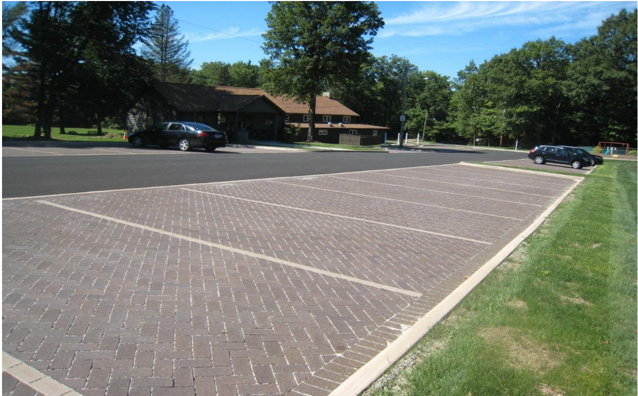
Permeable pavers at Centerville Mills Park reduce runoff volume and pollution from the parking lot.
